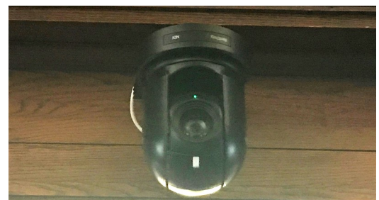
Cameras-three total-powered over ethernet rest beneath the ledge just below the balcony. They are controlled remotely.
