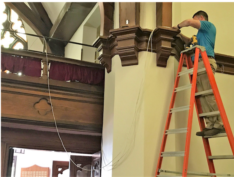
Jerry from Technicom carefully strings ethernet cable from the server room upstairs along a ledge in the Sanctuary.
